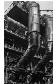
Steelworks plumbing Accepted Grahame Wilson
