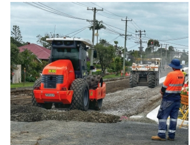
Repaving road Accepted Wanda Amos
